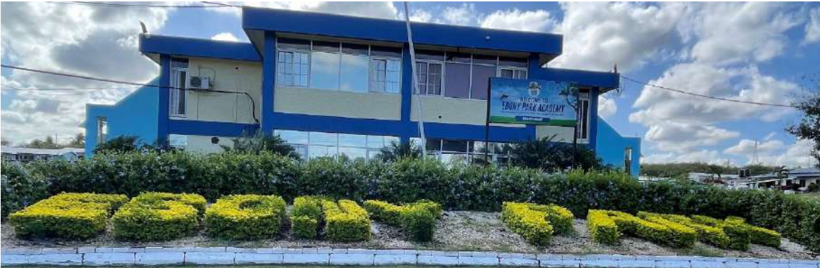
EBONY PARK ACADEMY AGRO-PROCESSING PLANT
