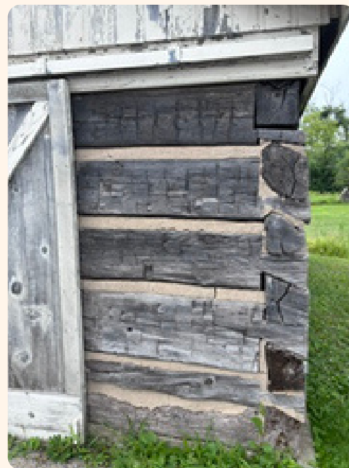
CLARK HOUSE SHED RESTORATION SIDE
