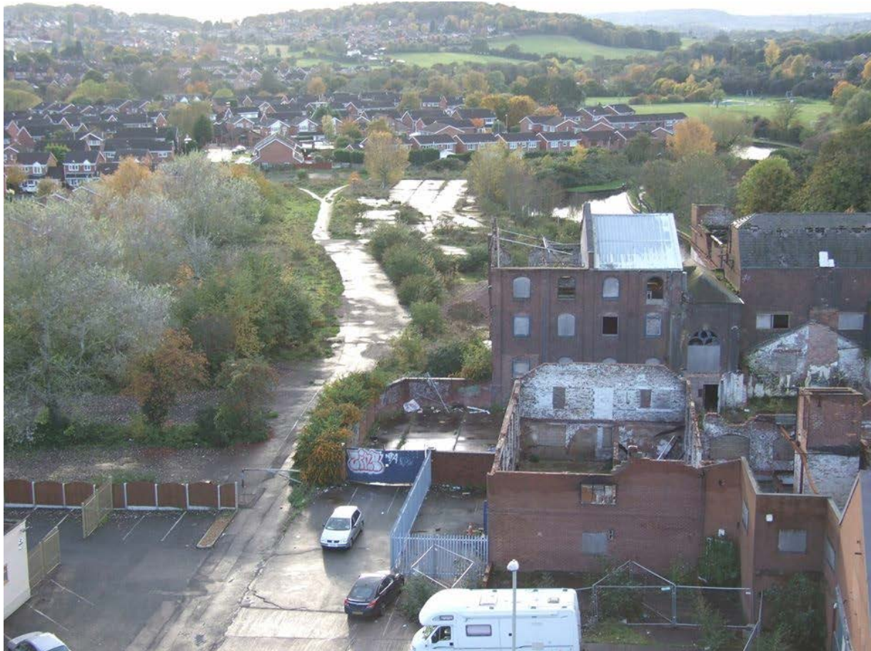
The derelict White House Cone site in Wordsley
