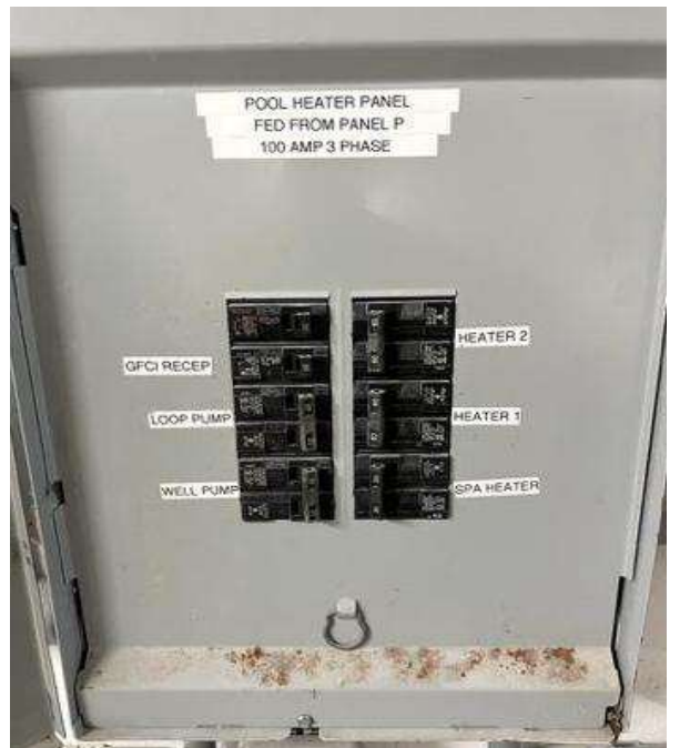
Picture #28 Pool panel is in good condition.
