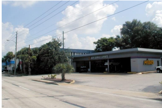
Property with two closely spaced driveway openings
