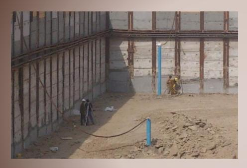
Dewatering means "the separation of water from the soil," or perhaps "taking the water out of the particular construction problem completely."
