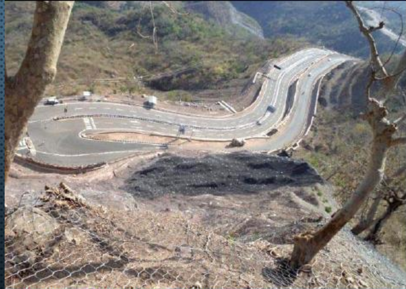
Steelgrid BO during installation
