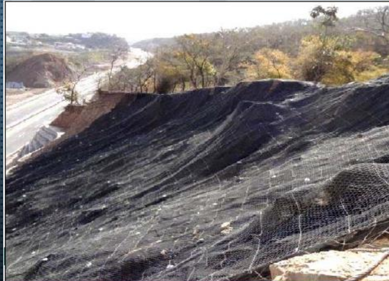
MacMat R used in conjunction with Steelgrid BO in places
