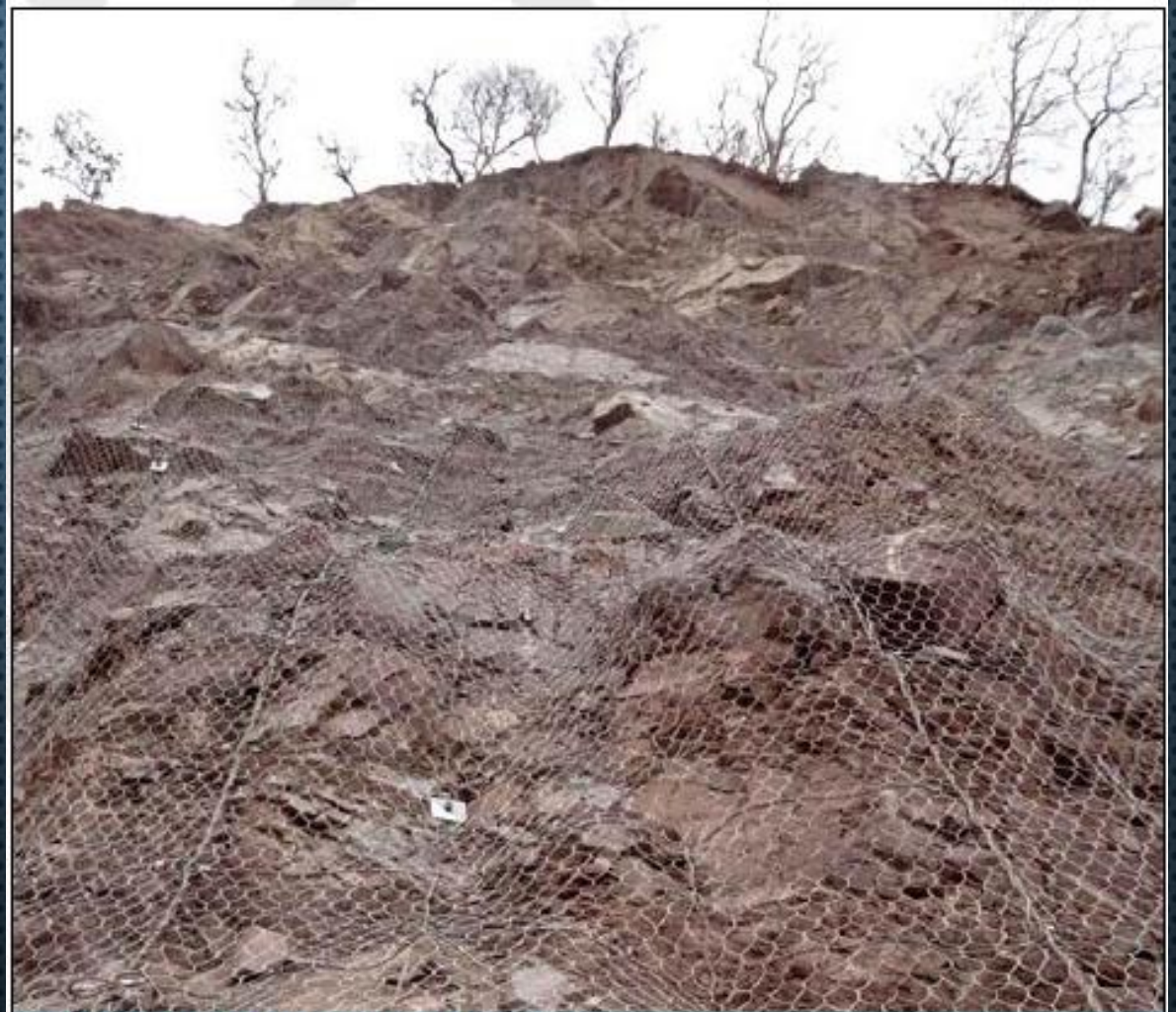
Steelgrid BO during installation
