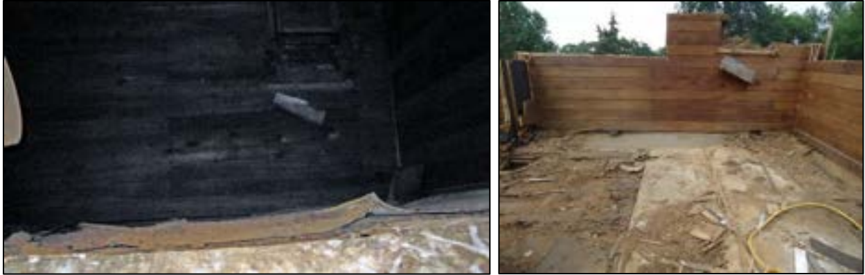
Sheets of galvanized metal with standing seams covered the tank room floor. These photographs were taken from the tank room doorway facing north before (left) and during (right) disassembly. (Photographs by Paul Bergson, left, and Curt Richter, right)
