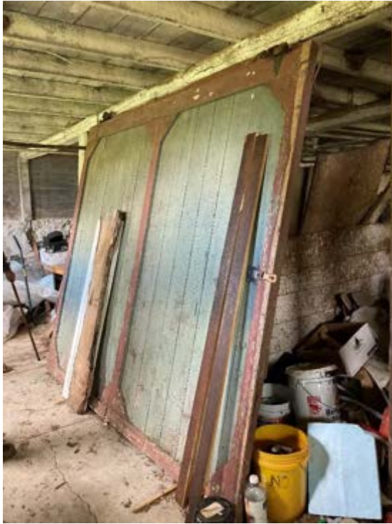
Figure 3 – One of the west barn doors.
