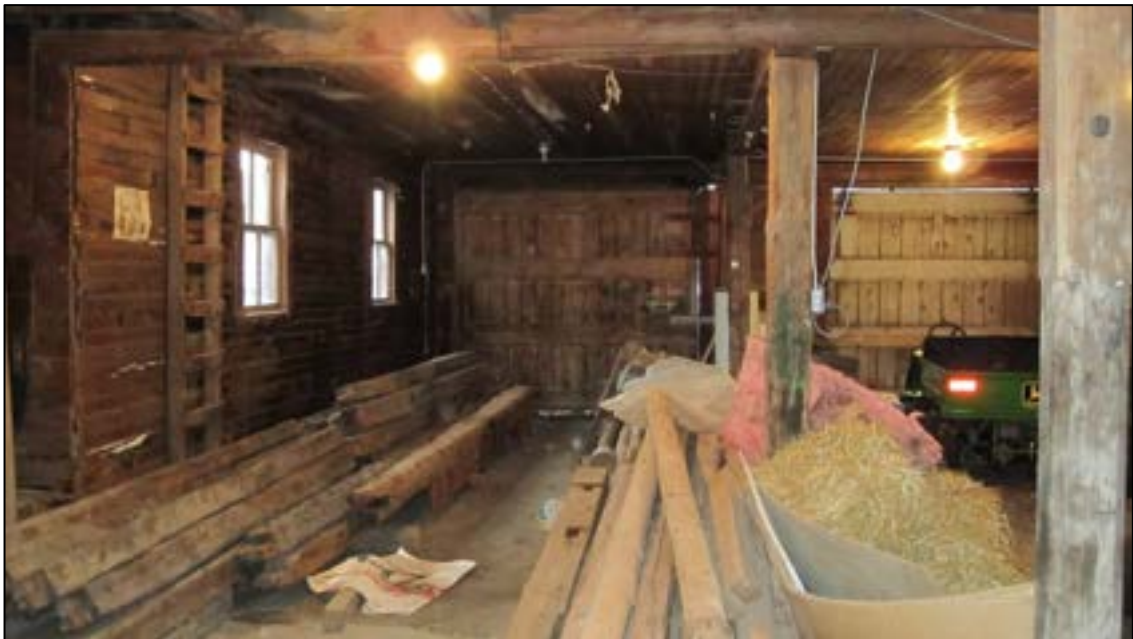
Interior of west section. (Paul Bergson photographs) Top: Second floor. Bottom: First floor.
