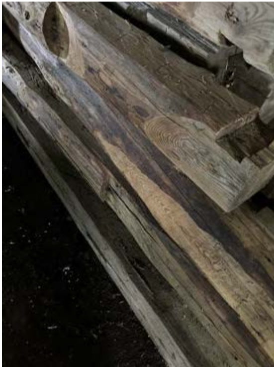
Figure 5 – Timber members showing hand-hewn notches.
