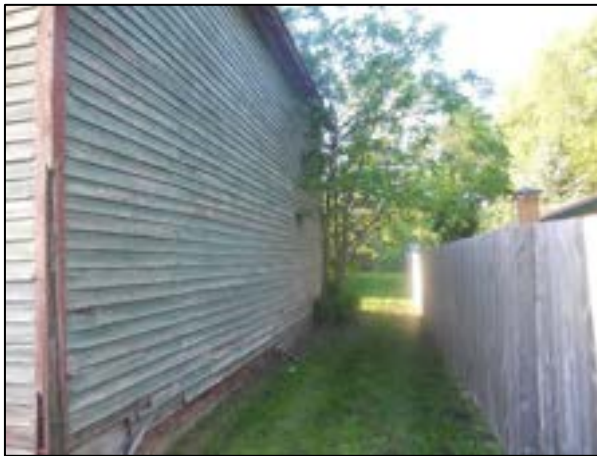
Filled-in openings on the east wall before (top) and after (center) the interior sheathing was removed. The exterior clapboard (bottom) showed no evidence of the openings. (Photographs from Two Pines, top; Curt Richter, center and bottom)
