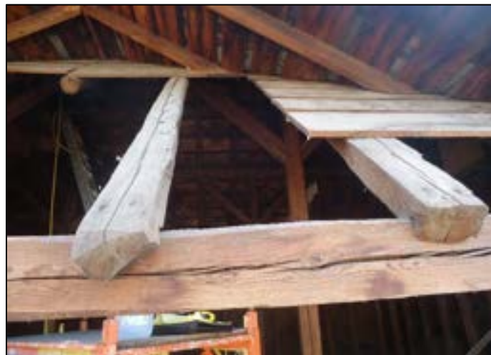
Where the east and west sections intersect, the rafter tails of the east roof were on the interior. They were trimmed differently than the rafter tails exposed on the exterior. (Curt Richter, photographer)
