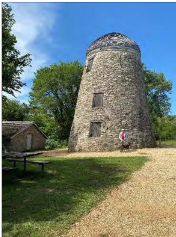
The 1864 Seppman Mill, a stone structure at Minnesota State Park near Mankato, is a good example of a European-style tower gristmill, although its arms are not extant.
