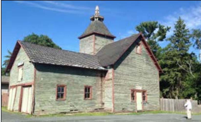
Photographs before barn was disassembled.
