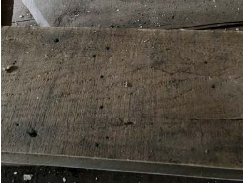
Figure 1 – Dimension lumber barn member showing machine milled saw marks.
