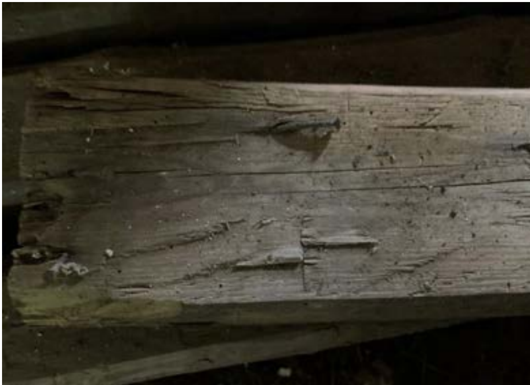
Figure 2 – Timber barn member showing hand-hewn adze marks.
