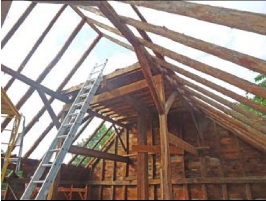
Left: The structure supporting the tank room was visible when the barn was disassembled. (Curt Richter photograph)
