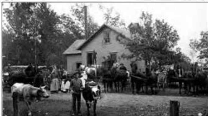
Top: The Kineth Farm Barn (2006) Island County, Washington (HABS No. WA-248-A) Center: Littleton (Kingen) Round Barn, Hancock County, Indiana (HABS No. IN-159) Bottom: Scandia Creamery, 1894 (Minnesota Historical Society)
