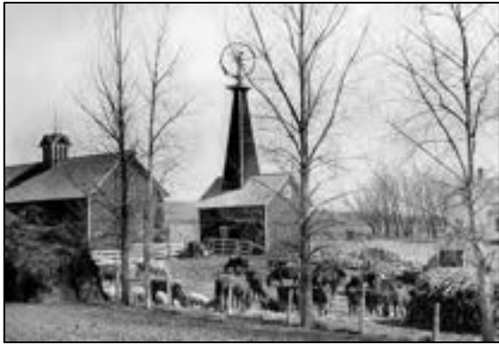
This circa 1910 windmill was mounted on a barn and furnished power for sawing and grinding as well as pumping. (Minnesota Historical Society)
