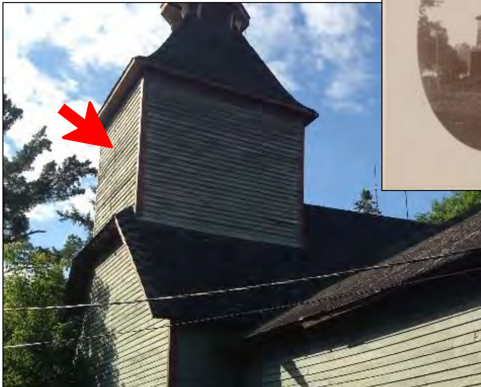
Below: A cable (perhaps from a lightning rod; highlighted with an arrow) bisects the north (left) side of the tower, but the clapboards show no sign of an opening.
