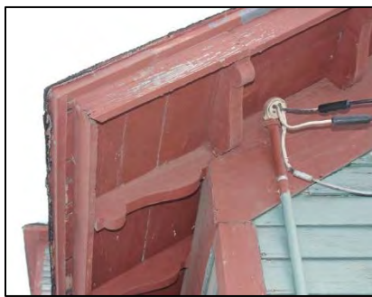
Detail views of curved purlin brackets (above, right, and center), exposed rafter tails (below), and tower brackets (bottom right). (Curt Richter and Susan Rodsjo photographs)
