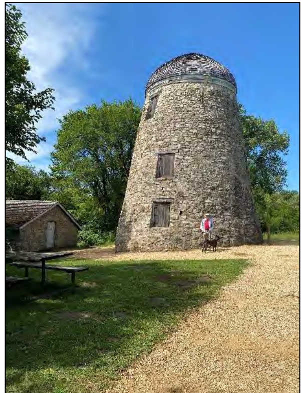
The 1864 Seppman Mill, a stone structure at Minneopa State Park near Mankato, is a good example of a European-style tower gristmill, although its arms are not extant.
