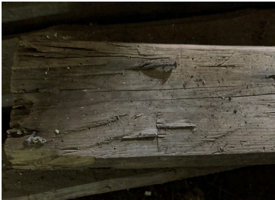
Figure 2 – Timber barn member showing hand-hewn adze marks.
