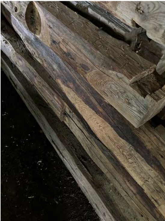
Figure 5 – Timber members showing hand-hewn notches.
