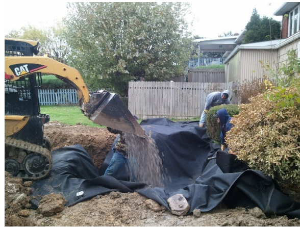
Separate stone fill from soil with straw layers or fabric
