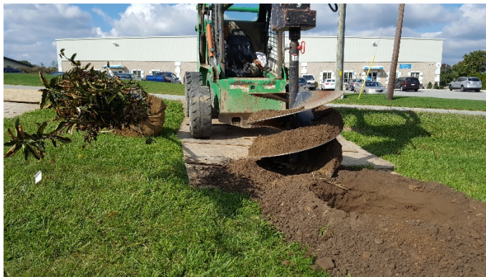
Plywood sheets protect lawn from compaction
