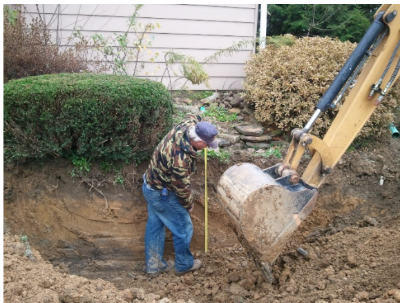
Excavate a drywell at least 10' from foundation
