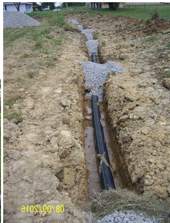
Perforated pipe covered in stone with straw separation layers
