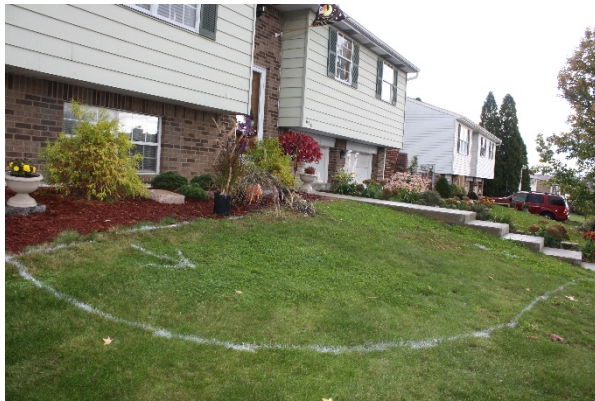
Mark rain garden location to avoid utilities
