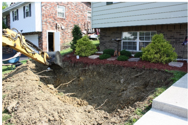
Excavate rain garden at least 10' from foundation
