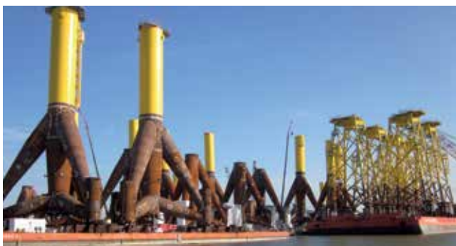
Wind turbine construction
