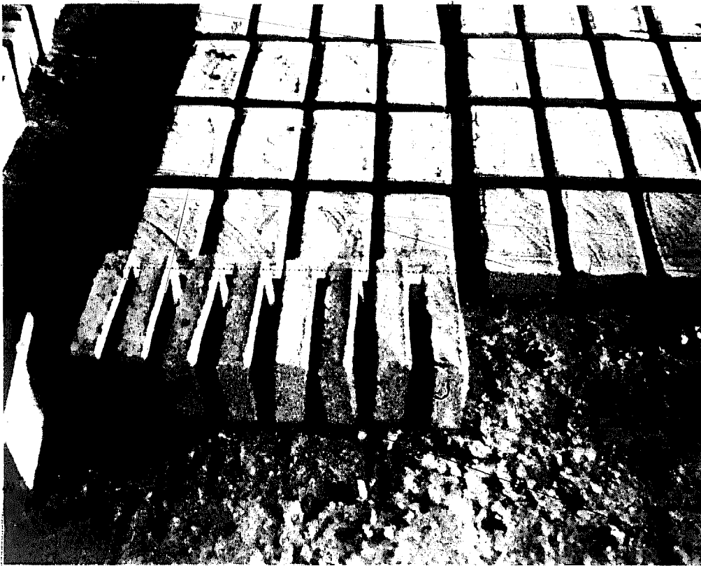
After drying the bricks are fettled to improve shape
