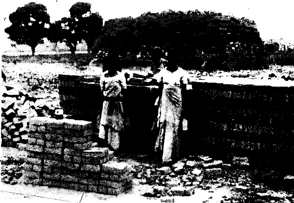
Wood-fired clamp under construction by lady brickmakers. Lack of suitable hand trucks leads to excessive carrying. Some shape defects can be seen in bricks in the foreground
