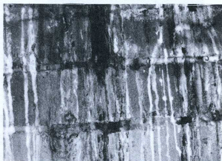
Figure 1-3. A close-up of a chimney with possibly terminal creosote damage. The acidic creosote has eaten away at the mortar joints, making them porous and a fire hazard.
