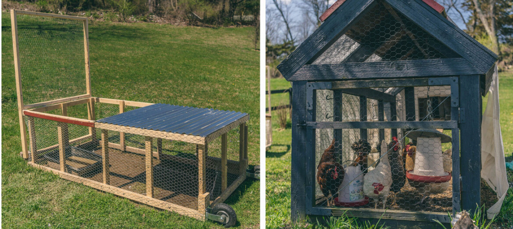
A movable tractor trailer was built for the ducks, and the chickens were placed in the smaller coop in the front of the house temporarily during construction of the new, larger run.
