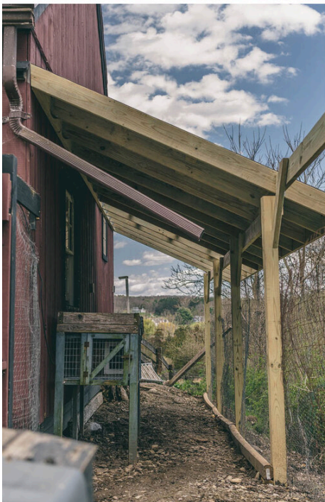
A lean-to was attached to the barn to provide shade and protect the flock from rain and snow. There will be doors at either end of the run. Finally, the pond area will be placed another 16ft to the left (picture-bottom left)
