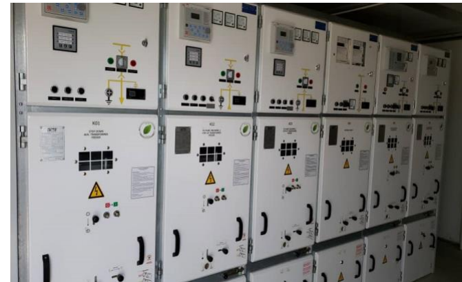
Figure 2: LV Panels & Components
