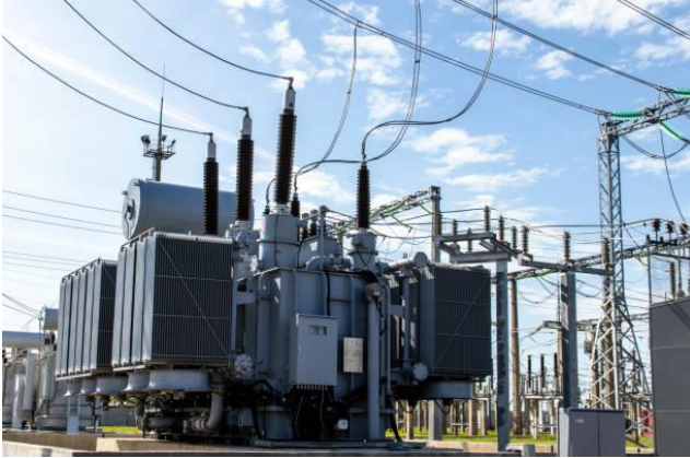
Figure 7: Power Transformers
