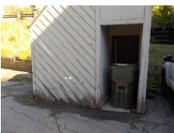
**Description:** Common area wood dumpster enclosures, with an asphalt shingle roof.
