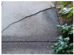
**Description:** Concrete sidewalks and patios, cast in place, reinforced concrete slab with a broom finish.
