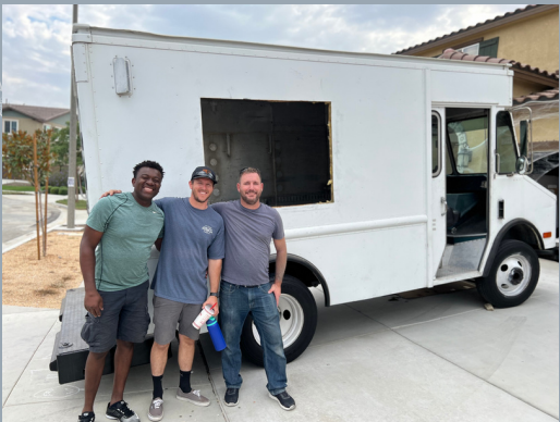
Francklin, Steven, & Brandon successfully cut out the hole for the serving window!
