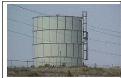
Water Storage Tank North of Burlington
