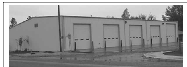
Big Horn Fire District #4 Fire Hall, Burlington
