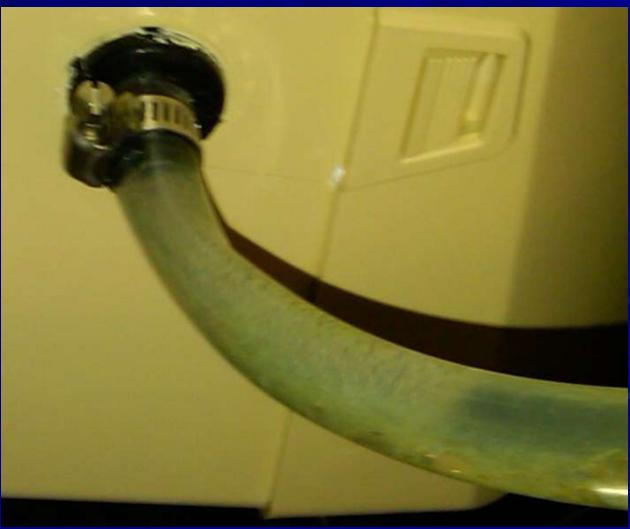
A small air leak around the drainage hose attachment was creating bubbles in the waste water which was backing up into the humidifier
