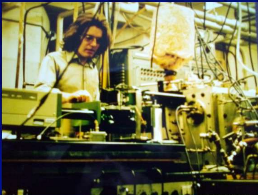
Fall 1973: Basement Building 4 Resonance enhanced laser ionization mass spectrometry of four aromatic molecules Charles T. Rettner , John H. Brophy
