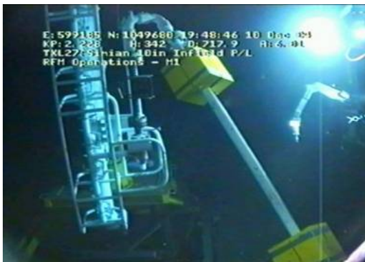
Figure 11 – RFM loading arm stabbed in
