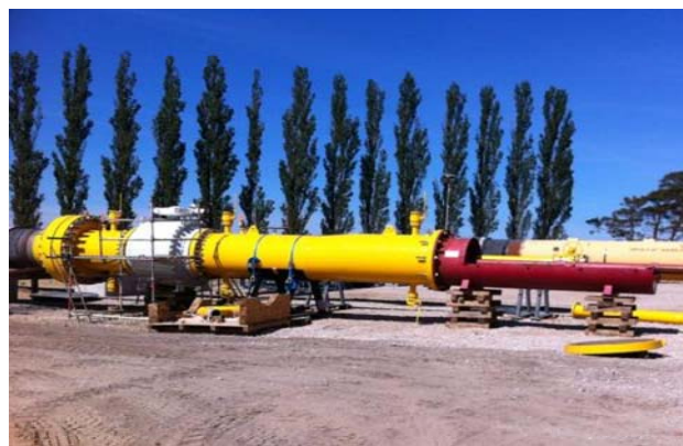
Fig. 10: Temporary Pig Trap: German Landfall
