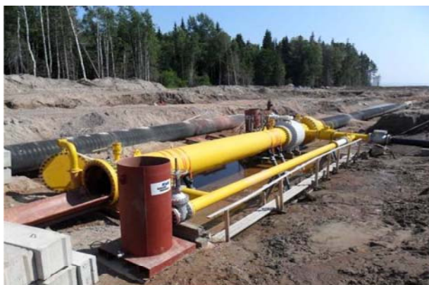
Fig. 9: Temporary Pig Trap: Russian Landfall
