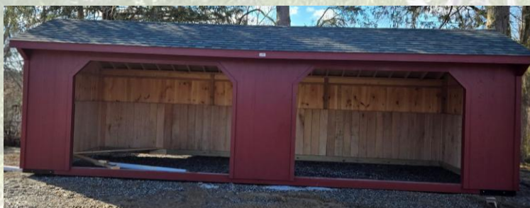
New Verizon Hay Storage Shed
