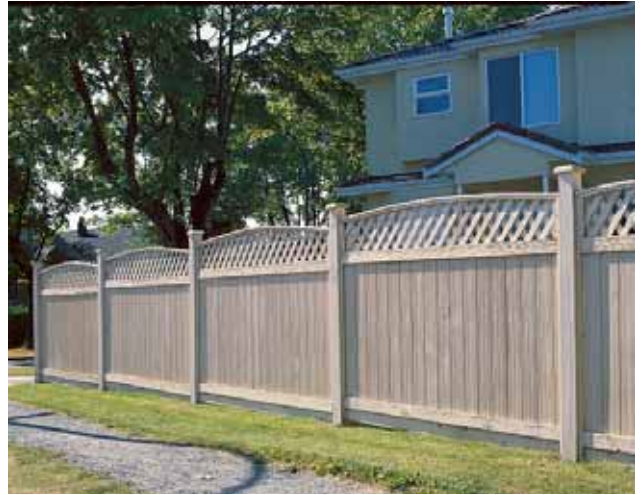
The graceful curve of the top rail and latticework reduce the scale of this solid board fence.
