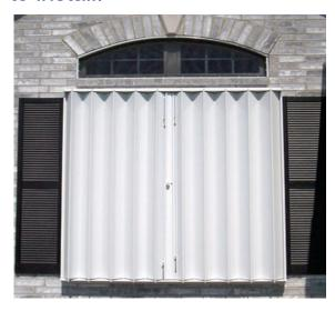
Our Accordion shutters are easy to install, safe and economical. The StormSecure systems are extremely weather resistant and excellent for indoor and outdoor storm and security applications. It has a nice low-profile when open.
