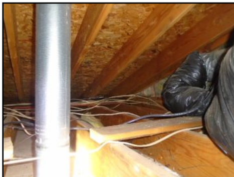
(Garage Attic) Wiring should be secured to the framing
