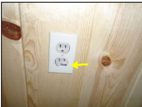
Master Bedroom Outlet Broken Recommend replacement.
