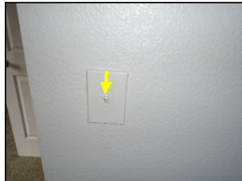
Master Bedroom Switch and Plate Covered in Paint
