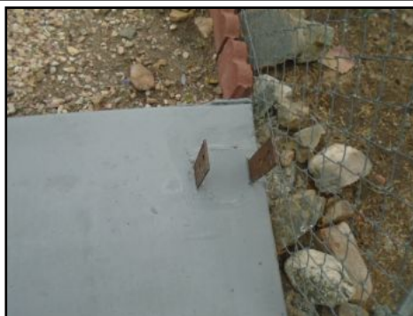
Support Bracket Could be a tripping Hazard. Recommend a Decorative Cover for Safety and Covers Eye Sore
