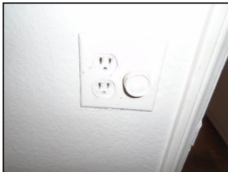
Outlet is covered with Paint as with alot of the Outlets in the House
