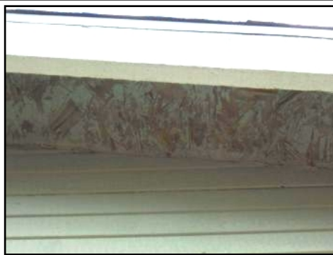
Unfinished Material up in the Eaves. Recommend Further Evaluation by a Handyman.
