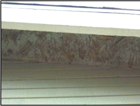
Unfinished Material up in the Eaves. Recommend Further Evaluation by a Handyman.
