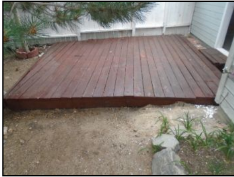
Septic Tank is Located under the Back Deck.
