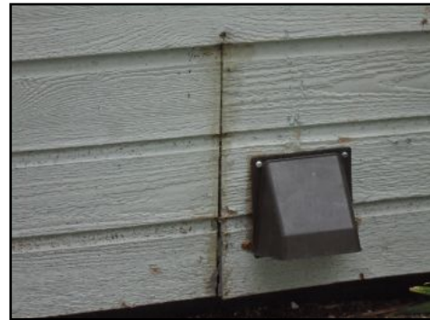
Seal all gaps and Cracks
