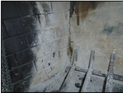
Fire Box has some big cracks in it. Recommend further evaluation by a Chimney Contractor to see if this is Okay to have the insert just put in or anything needs to be done first.
