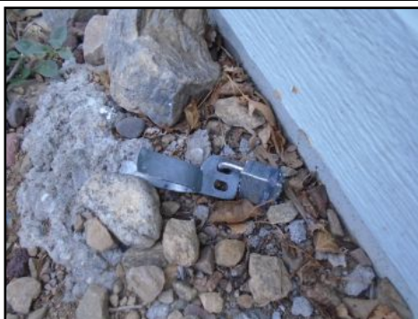
Gate Latch is off the Gate. (Side of the Garage By Electrical Main Panel)
