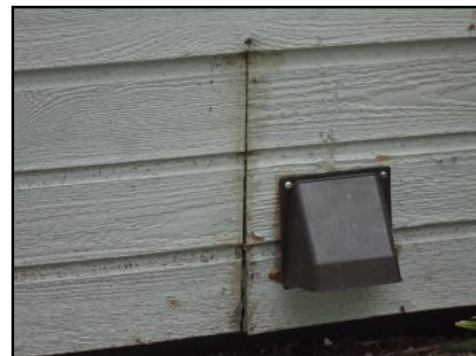
Seal all gaps and Cracks
