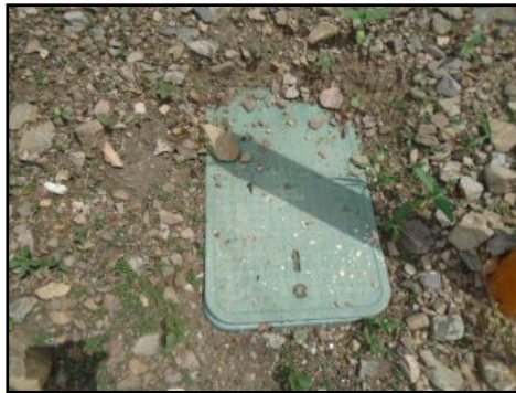
City Water Main Valve & Meter
