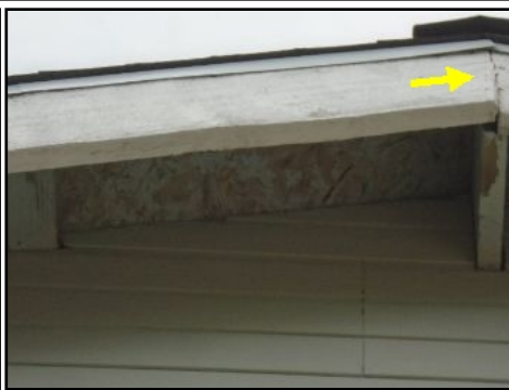
Facia Board is Twisting. Secure or replace with a new pre sealed and painted board to assure sealing.
