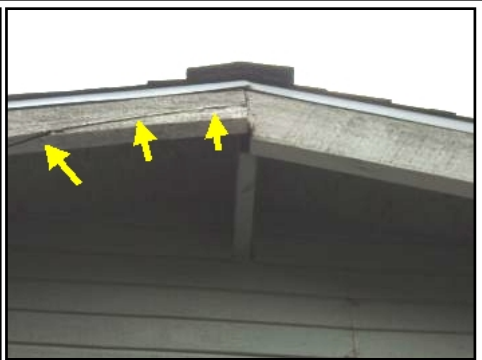
Facia Bard is Cracked and Twisted. Recommend Further Evaluation by a Handyman
