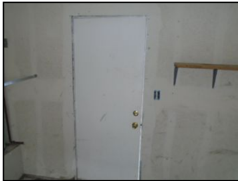
Garage to Outside Door
