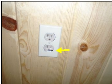
Master Bedroom Outlet Broken Recommend replacement.
