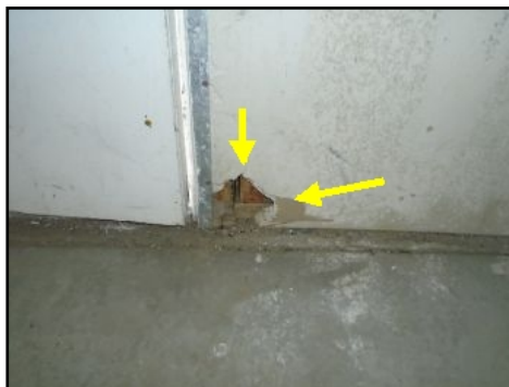
Hole in Garage Wall
