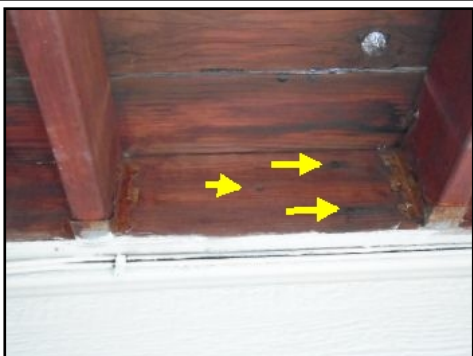
No Lag Bolts or Screws. For Safety reasons you might think about added at least Lag Screws to help support.
