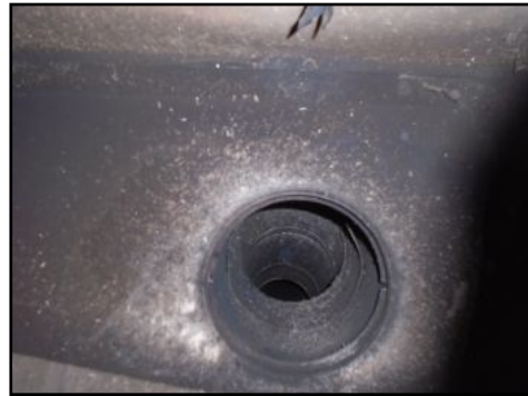
Flue appears to just be open with no Damper
