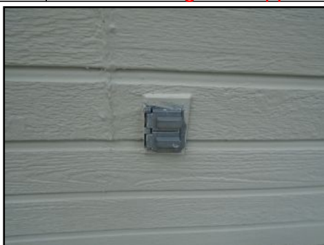
Outlet is dead (No Power). Recommend Further Evaluation by a Handyman or a Licensed Electrician.
