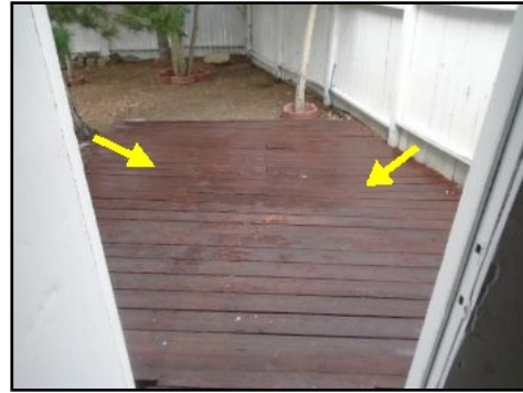
Out Garage Door and Under Back Deck
