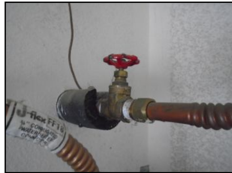
Supply Shut-Off for the Water Heater
