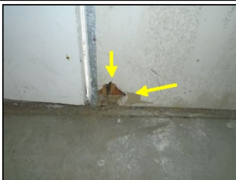
Hole in Garage Wall
