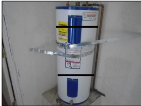
This Is One Strap and Done Incorrectly. Must 2 straps 1 at bottom 1/3 and one at top 1/3
