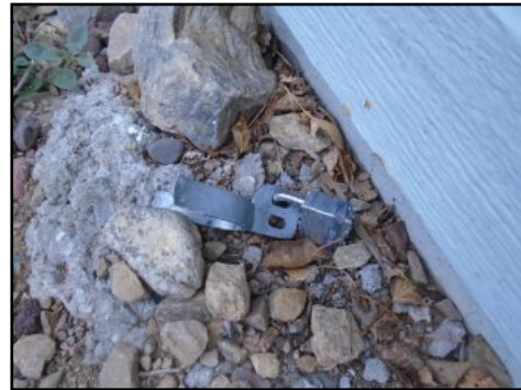
Gate Latch is off the Gate. (Side of the Garage By Electrical Main Panel)
