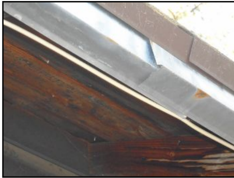
Flashing is separating. Recommend sealing,
