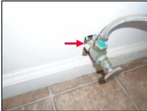
Seal Hole around the Pipe
