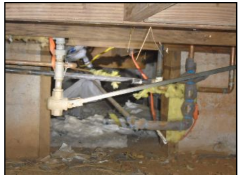
Entrance to the Crawlspace has been almost completely blocked with plumbing. Could not Access
