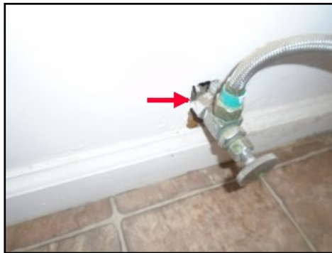
Seal Hole around the Pipe
