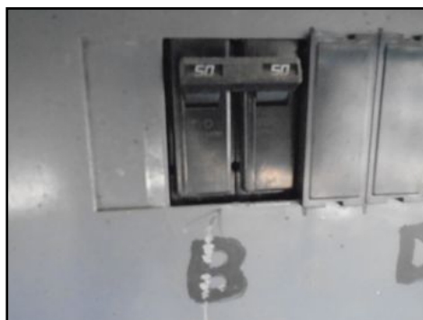
Building "B" Main Breaker is 50 Amp
