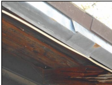
Flashing is separating. Recommend sealing,
