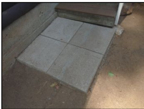
Landing at the Back deck. Could be a Tripping Hazard
