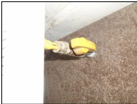
Gas Valve For Living Room Wall Heater
