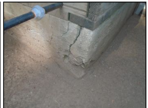
Crack In Foundation wall
