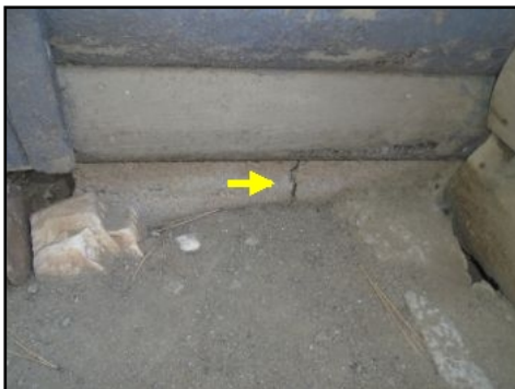
Crack in Wall
