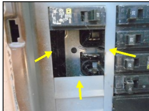
Sub Panel For "A" has 2 open spots.
