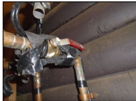
Shut Off Valve for the Water Heater Supply.
