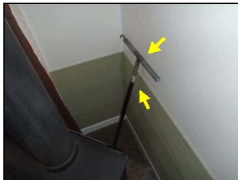
Key For Outside Stop &amp; Waste
