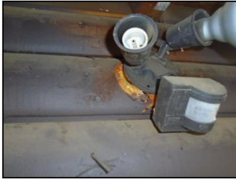
Not the proper way to install & Seal a Light Fixture
