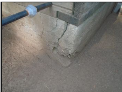
Crack In Foundation wall
