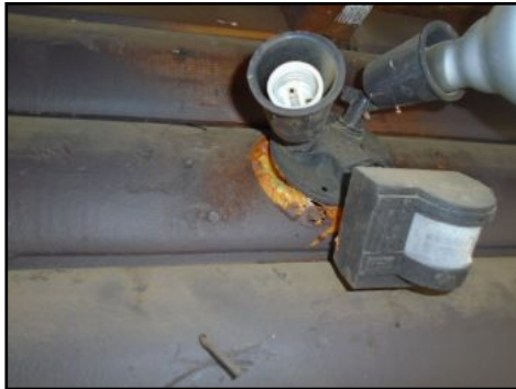
Not the proper way to install &amp; Seal a Light Fixture
