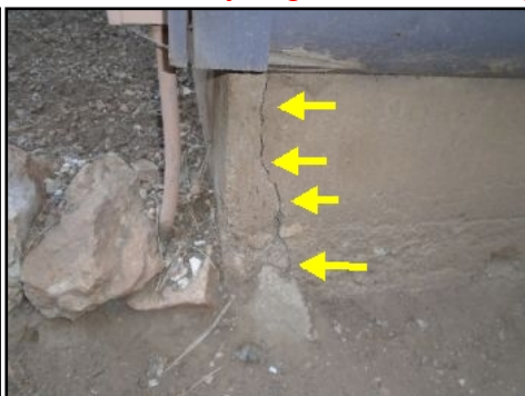
Crack in Foundation Wall
