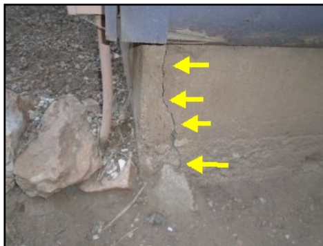
Crack in Foundation Wall
