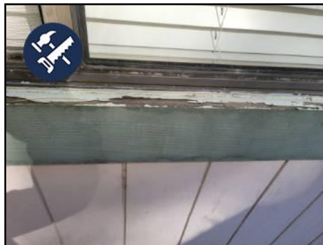
South Side--Peeling Paint & Bare Wood Observed
