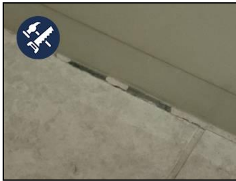
Bathroom#2 Caulking Needed
