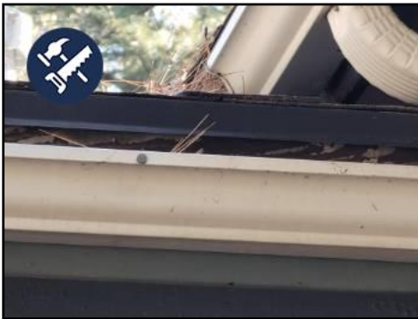
Gutters are filled with Pine Needles. These should be cleared.
