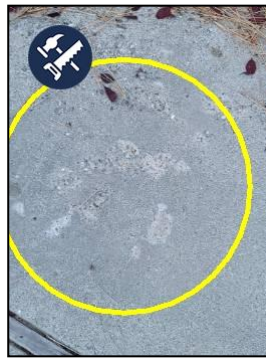
Spalling on the Driveway
