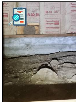
Efflorescence Observed
