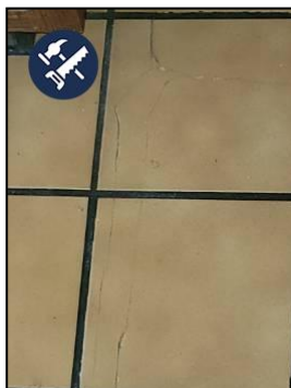
Cracks in the Kitchen Tile Flooring
