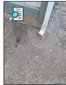
Southeast Corner--Monitor the area and see if water builds up here at the Foundation wall, if it does need to make it move along as too not continually soak the Foundation Wall
