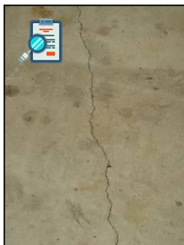
Crack in the Garage Flooring
