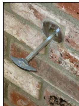
Gas Log Lighter Assist System-- Gas Valve & Key
