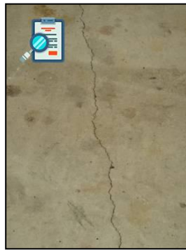
Crack in the Garage Flooring
