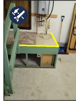
Not Actually required but recommend railing around the Landing Deck
