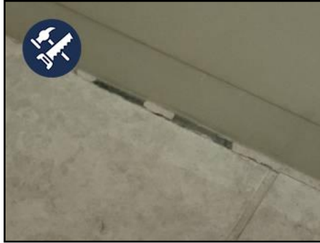
Bathroom#2 Caulking Needed
