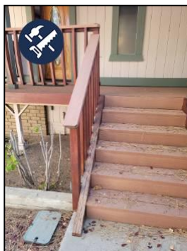
Handrail is Loose
