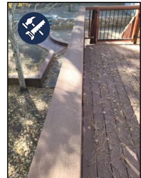
Rear Deck Railing is Loose
