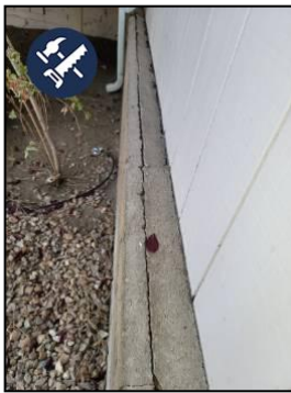
Cracked across the top of the brick veneer
