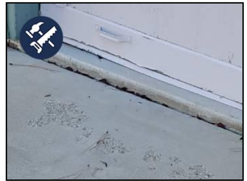
Possible tripping hazard going in garage
