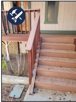
Handrail is Loose
