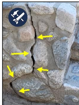
Rear Yard Major Crack in the Stone Veneer
