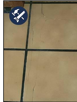
Cracks in the Kitchen Tile Flooring
