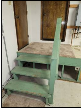
Handrail is a Little loose
