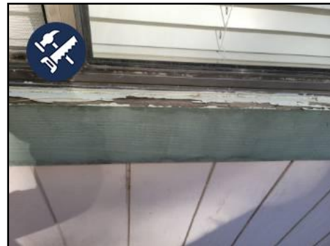
South Side--Peeling Paint & Bare Wood Observed
