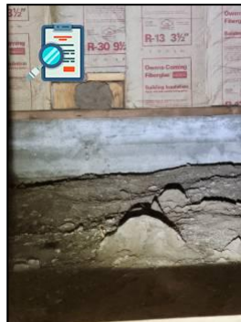
Efflorescence Observed
