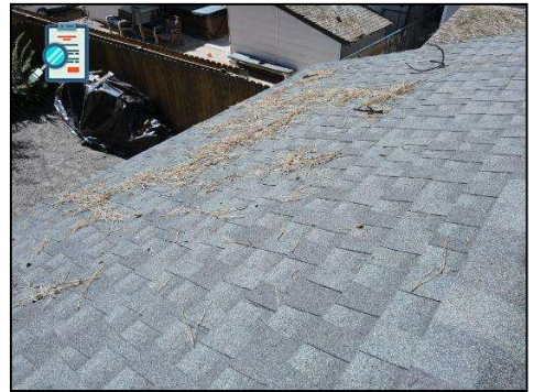
Clear Tree Debris Whenever Possible.
