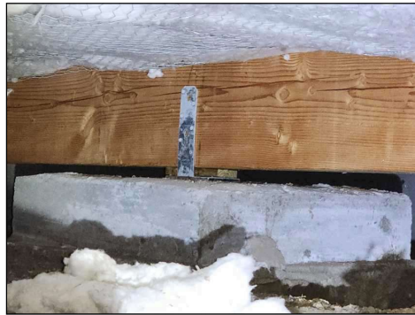
Concrete block/wood piers support floor above.
