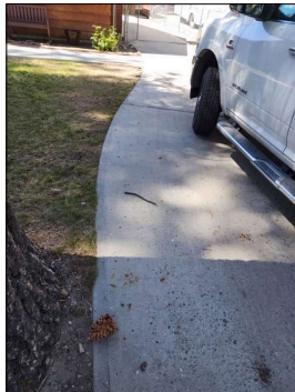
North Side Concrete Driveway.
