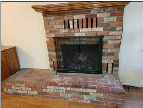
Living Room--Recommend having Fireplace Fully Inspected and Cleaned by a Chimney Specialist Annually
