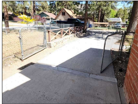
No Apparent Issues with the Gates. West Side.
