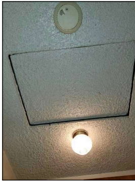
Access at hallway ceiling.
