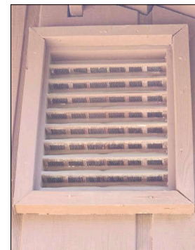
Vent screens noted as functional. South Side.
