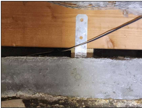
Concrete block/wood piers support floor above.
