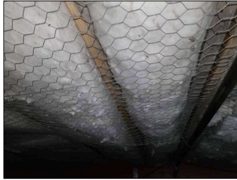
No Apparent Issues with the Insulation.
