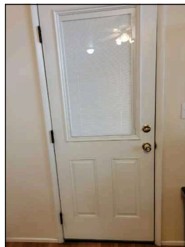
Rear Entry Door
