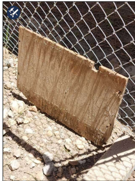
Entry Door is a Riddled piece of Plywood and should be replaced.
