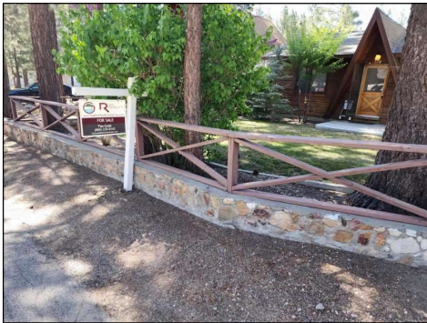
No Apparent Issues with the Fencing. North Side.
