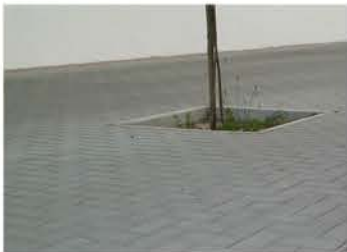
Interlocking "Holanda" con- crete block paving in entrance areas
