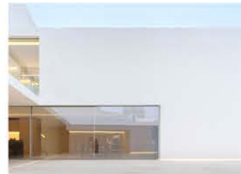
Exterior wall rendering with waterproof mortar, smooth troweled finish | White color
