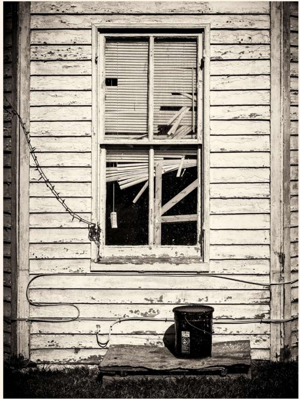
Derelict window A work in progress
