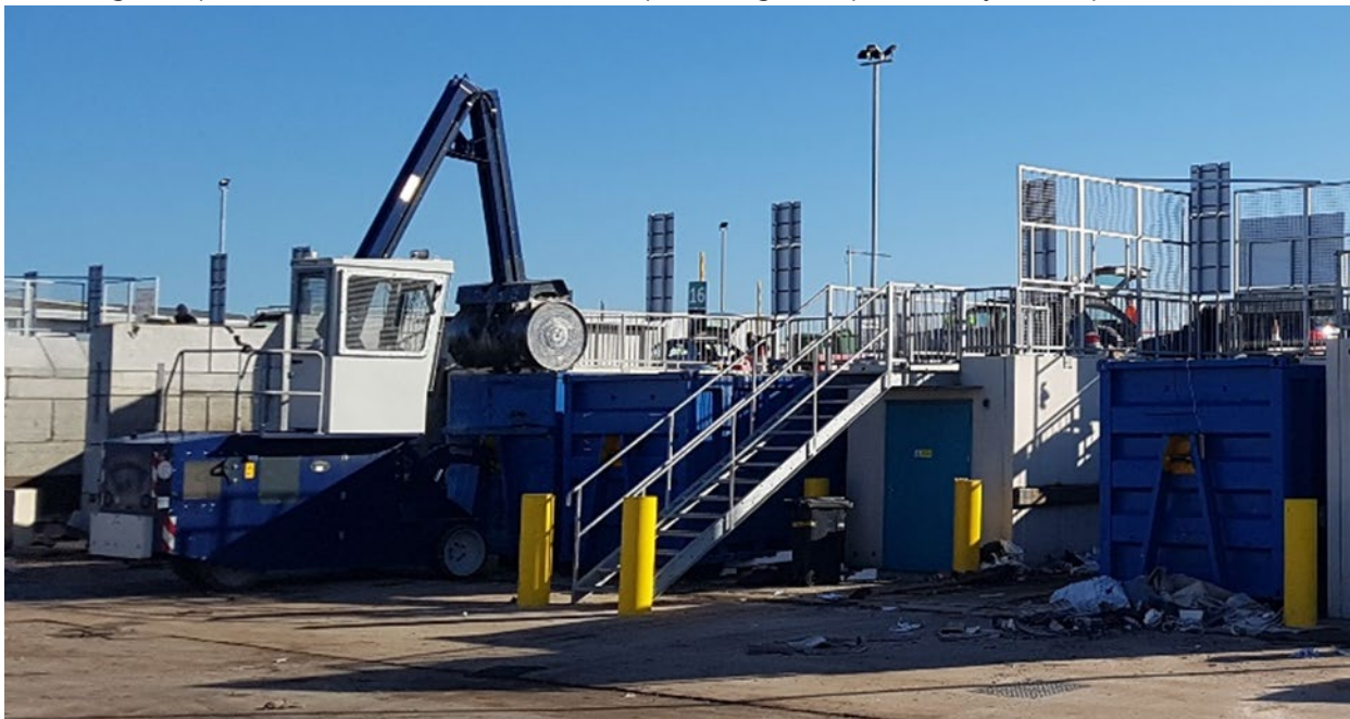
Figure 2 Skips for segregated materials and machinery to compact the content
