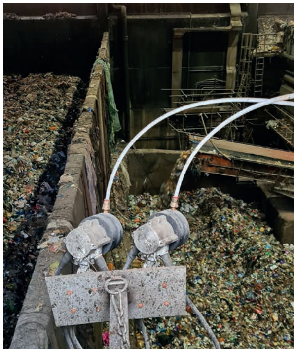
◀ Figure 3. Two FLS-IR3 detectors looking into a pit of partially processed solid waste.
