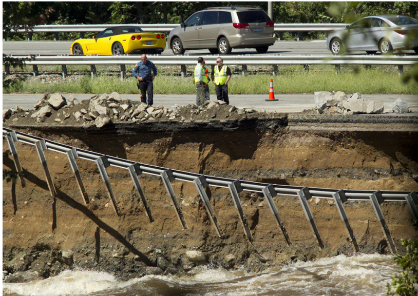
Figure 18 Collapsed shoulder of I-287 in Boonton, NJ on August 29, 2011. Steve Hockstein for the Star Ledger.
