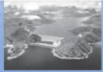
1978 Completion of High Island Scheme 281 mcm capacity
