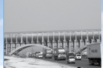
2003 Commissioning of 83km dedicated aqueduct for delivery of Dongjiang water
