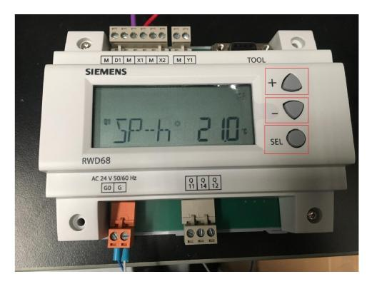
Press 'SEL' button, the number value will flash, adjust to desired value using + or – buttons. Press 'Sel' button to confirm selection.
