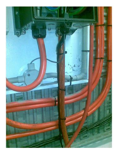
Good: A wide cable tray allows a reasonable distance to separate signal cables from power cables. Best practise is to keep 250mm clearance. Having the motor cable cross the supply cables at 90 degrees minimises any noise coupling.
