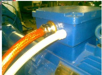
Left: This shows the minimum power wiring requirements for a Category 2 (Class A) installation. The strap is used to provide a good EMC bond between the motor cable and the drive, while the nylon glands maintain the IP55 rating. For Category 1 (Class-B) installations you must use EMC rated glands and the ferrite rings included with the drive. Note an additional earth bonding cable may be necessary.
