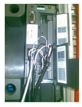
Right: Use the cable termination plate that is supplied with the drive to manage the separation of signal cables from power cables. This also allows for correct bonding of the shield when connecting sensors directly to the drive, e.g. when using the drive's internal PID loop to control cooling towers and stairwell pressurisation systems. Good: individual shielded signal cabling used to separate the analog inputs, digital inputs, and the status relay outputs.
