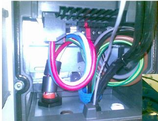
Good: Ferrite rings fitted & EMC rated glands used with shielded motor cable. Separate thermistor cabling. Bad: Cable loops and no bonding to the backplane using the metal straps provided with the drive.
