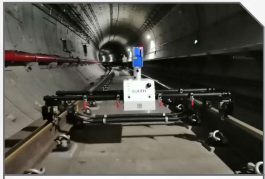
full inspection @ Guangzhou Metro Line 4 (tunnel clearance, diseases, etc.)
