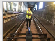
open-cut structure station
