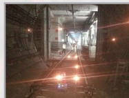
open-cut to shield structure part
