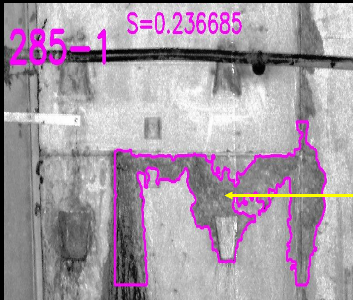
detected concrete falling-off in software
