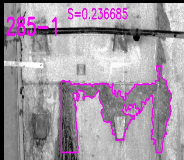
concrete falling-off
