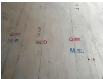
Layout for secondary structure construction
