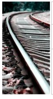
Gauge Measurement Measure the inner minimum distance (16mm below the surface) between the 2 tracks with gauge sensor.
