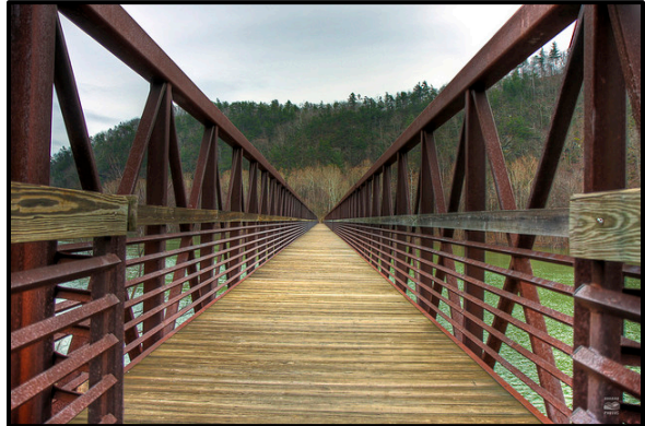
Figure 3 Bridge at Balcony Falls
