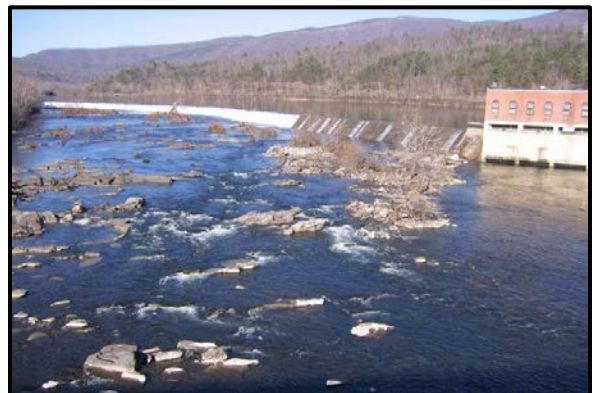
Figure 2 Balcony Falls Dam Near Town of Glasgow
