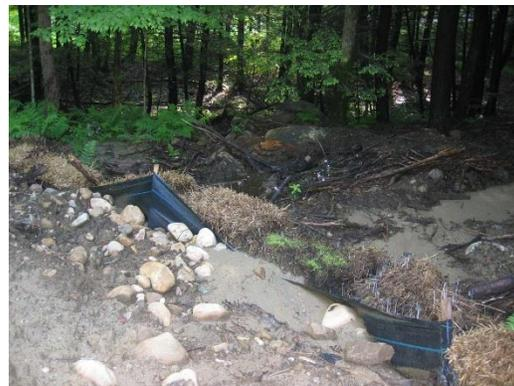
Sediment Overtopping the Silt Fence and Entering into Wetland
