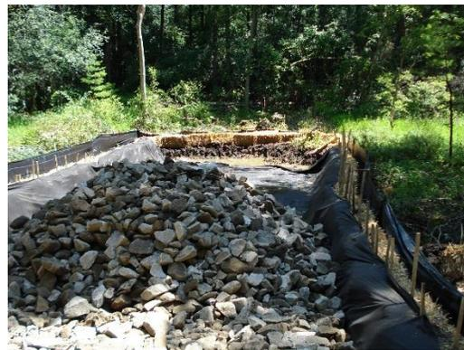
Trap Rock and Filter Fabric Placement through Wetland to Create an Unrestricted Flow
