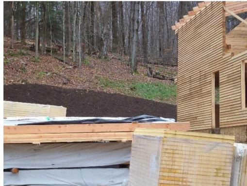
Stabilization of Slope with Geoweb, Topsoil, Seed and Mulch
