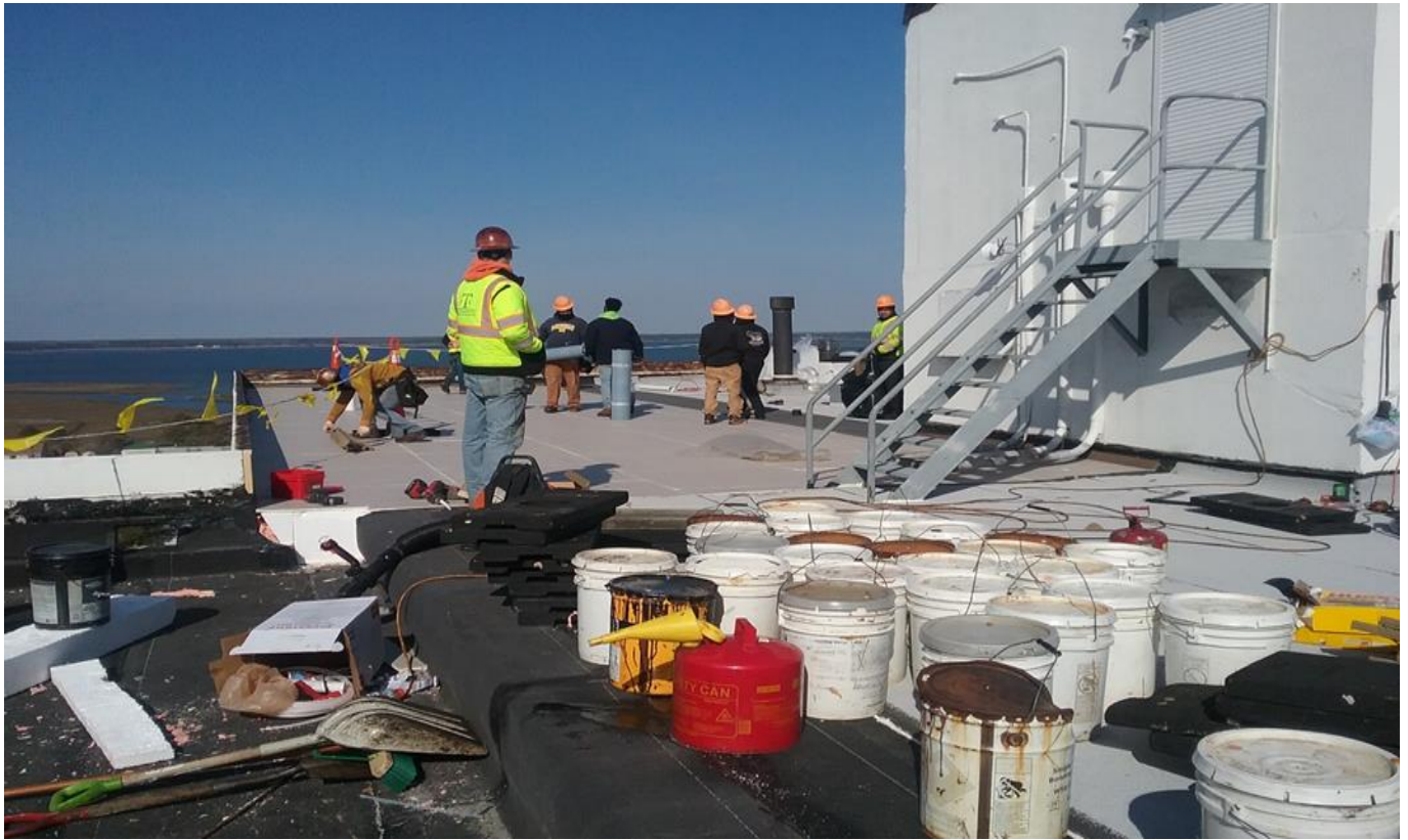
Once the blocks were in place, the final roofing materials were installed.
