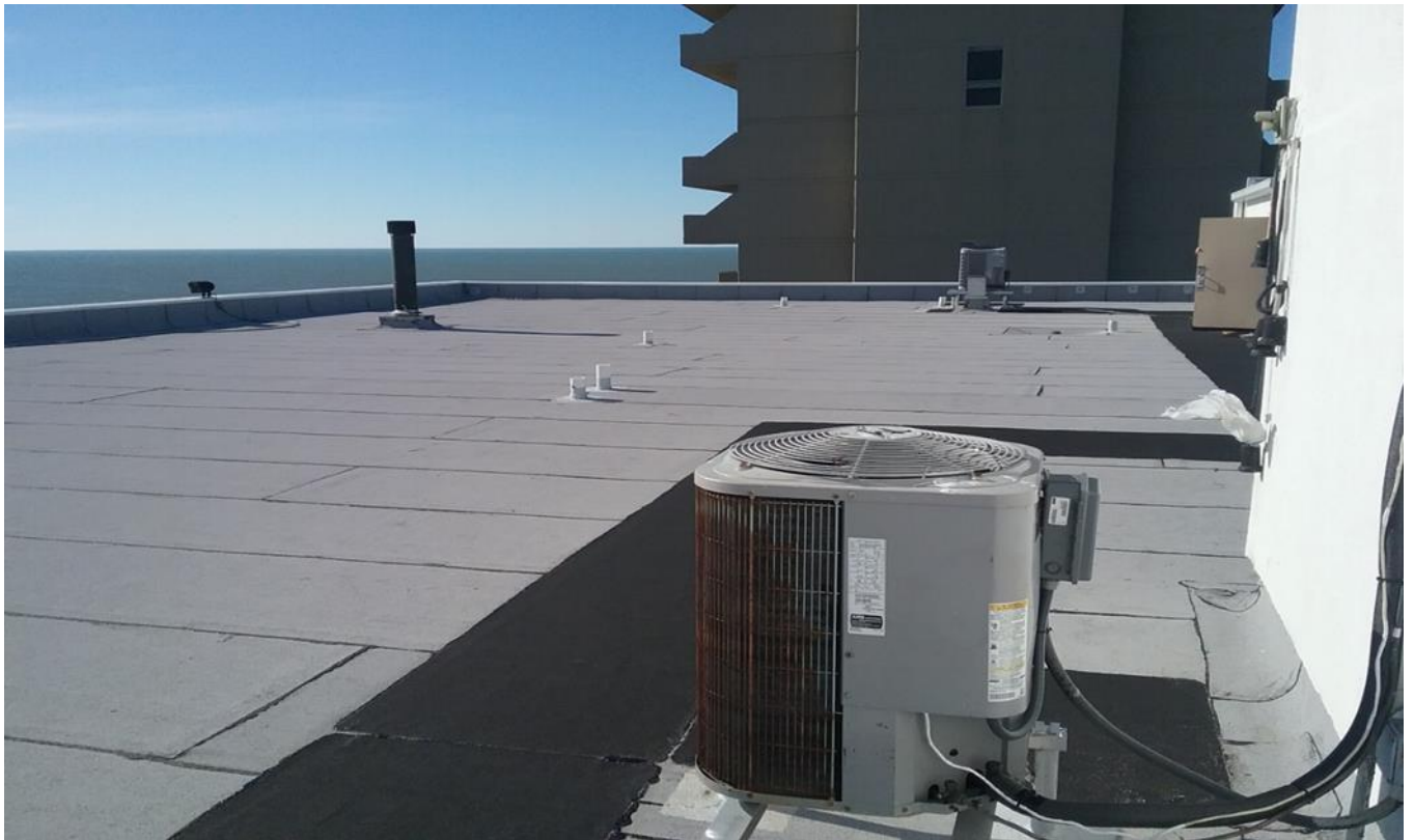
All of the other components on the roof also had to be reinstalled and/or modified for the difference in the thickness of the new roof in order to meet 2020 building codes.
