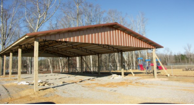
New 30' x 50' Pavilion erected January 2017 in Hamner Park (above)
