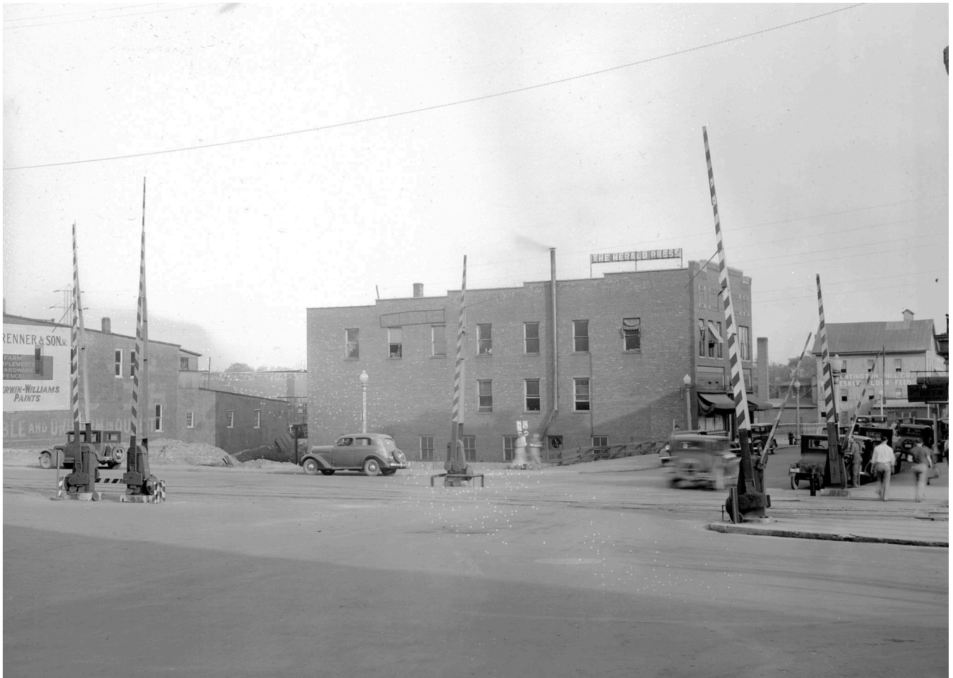
Looking south across the railroad tracks on Jefferson Street. In the center of the photo is the Huntington Herald-Press April 1936.
