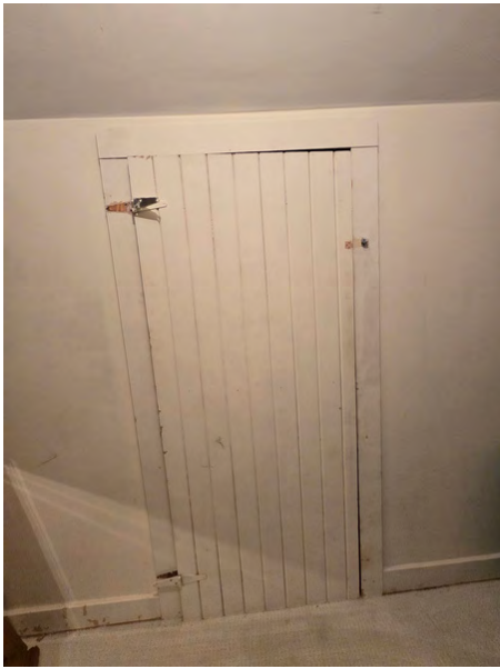
Door to eave attic storage on South end of home.
