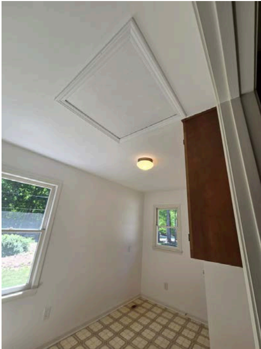
Attic Access (Scuttle Hole in Laundry Room.)
