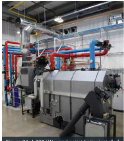
Figure 34. A 390 kW wood pellet boiler installed at Viessmann's Canadian Heaquarters. (Photo: Viessmann Manufacturing Company Inc.)
