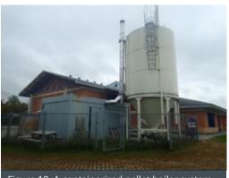
Figure 18. A containerized pellet boiler system with an agricultural silo for pellet storage used to heat a school. This type of containerized system can be used for cordwood, wood chip, and pellet boiler systems.
