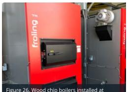
Figure 26. Wood chip boilers installed at Confederation College. Each boiler can provide 500 kW of baseload heat. Together, the boilers provide 85% of the space heating needs of the 400 000 square foot facility. (Photo: Biothermic)
