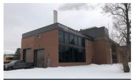
Figure 25. Wood chip boiler room and fuel storage facility at Confederation College. The garage door on the left leads to the on-site chip storage room. The door on the right leads to the boiler room. The system can be seen by passersby through the large windows. Wood chip boiler rooms do not need to be this large, but this boiler room was designed to accommodate tours and teaching. (Photo: Biothermic)
