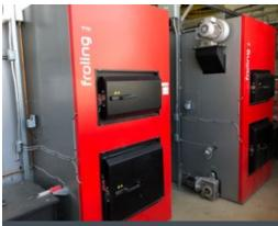
Figure 17. Wood chip boilers installed at Confederation College. Each boiler can provide 500 kW of baseload. These boilers provide 85% of the space heating needs of the 400 000 square foot facility. (Photo: Biothermic)
