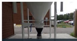
Figure 33. When the boiler's pellet hopper runs low, pellets are automatically delivered from the bulk storage silo shown above via vacuum hoses to refill the hopper.
