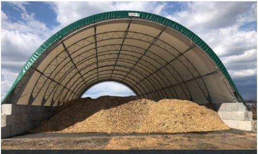
Figure 30. This bioheat wood chip production facility has an asphalt pad to eliminate dirt and sand contamination and keeps the chips covered to allow them to dry. It stores 1 000 oven-dry tonnes. (Photo: Biothermic)
