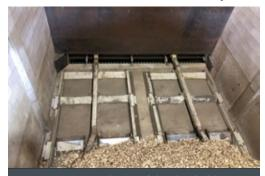
Figure 27. An aerial view of the chip holding room at Confederation College, engineered by Evergreen BioHeat. The scraper floor shown moves the chips along the room's length to a series of augers. (Photo: Biothermic)
