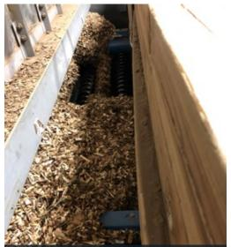
Figure 28. A series of augers automatically feed the chips to the boilers when there is a call for more chips from the boiler's control system. (Photo: Biothermic)
